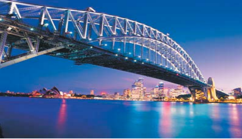
Sydney Harbour Bridge
